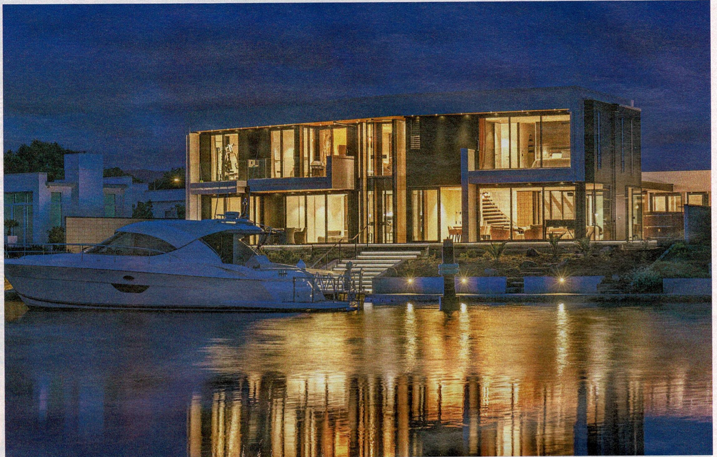
The 700sqm home includes 35 tonnes of structural steel and 760 individually cut blocks making up curved interior walls.
